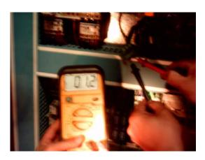
Disconnect motor cable and use ohmmeter to check the three legs. Every two legs should be even. If not even, problem is the motor. If even, the problem is the cable.
