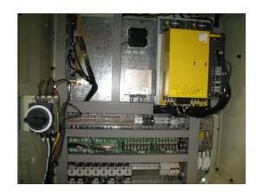
Output L1, L2, L3 (200V to CNC control) use meter check to make sure 200V
